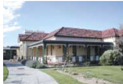
Existing facilities will be refurbished with state-of-the-art facilities
