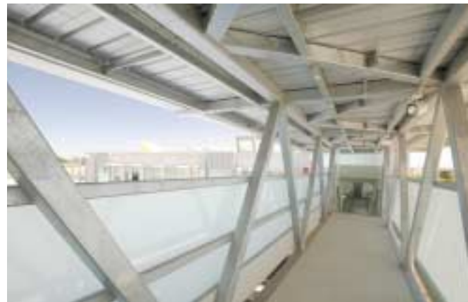
Interior view – Walkway
