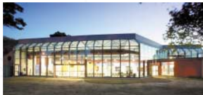
Broadmeadows Leisure Centre at night
