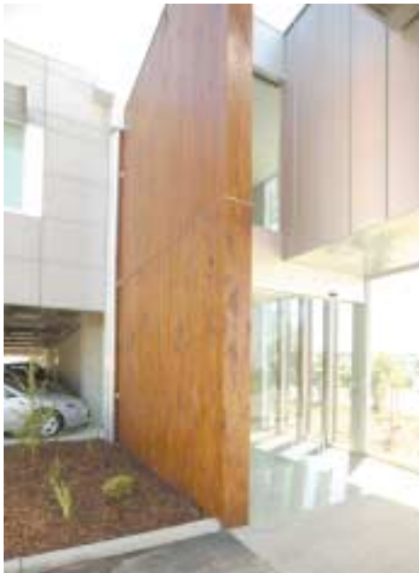
Completed Nufarm building
