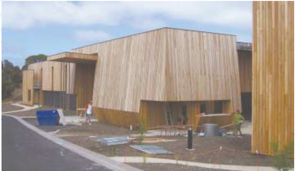
Finishing touches at Moonah Links Residential Lodges
