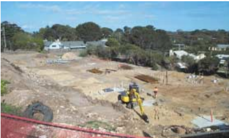
Excavation work at Delgany
