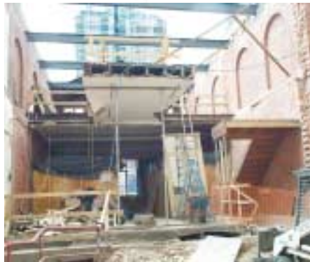
Current construction at 111 Little Lonsdale Street, Melbourne
