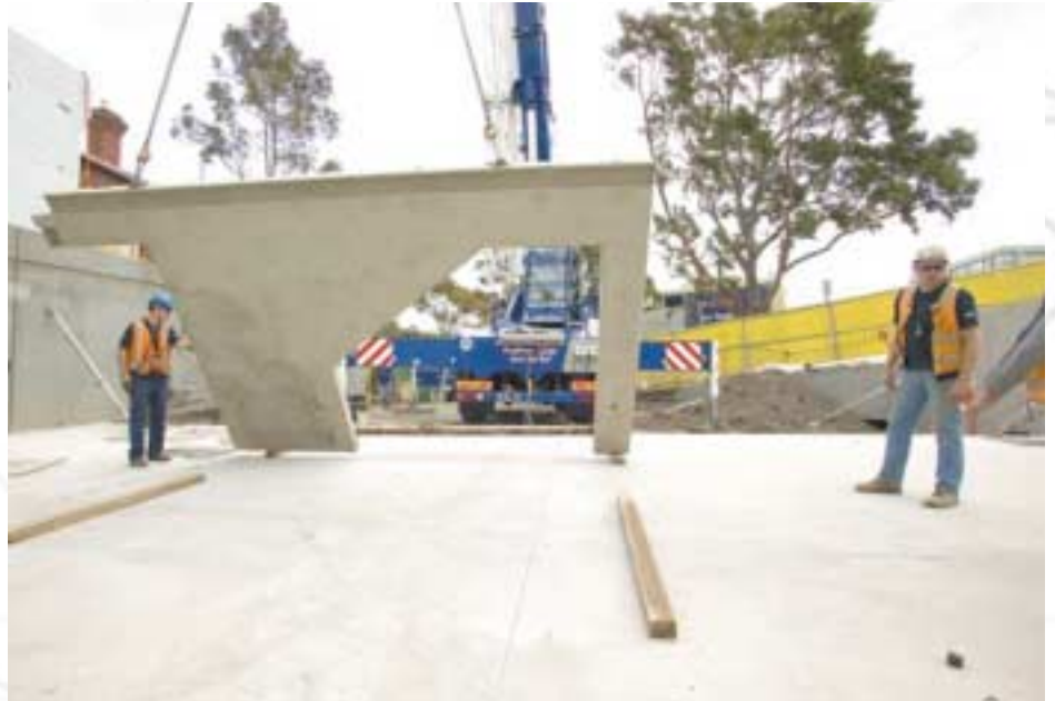
Early stages of construction at 56 Burwood Road
