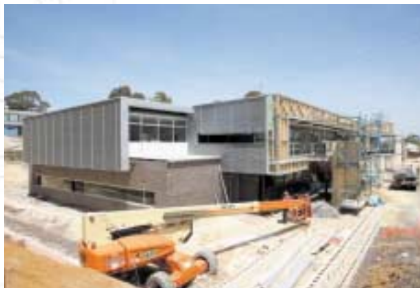
Construction progress during October
