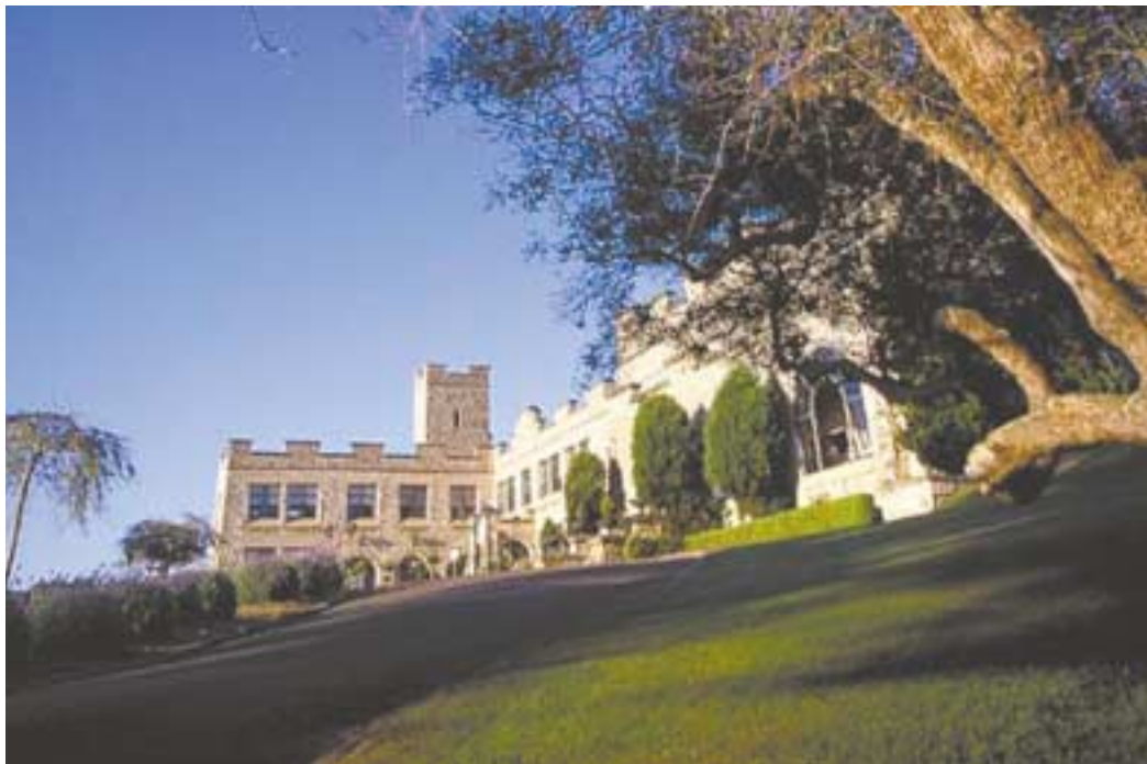
Exterior view – Delgany
